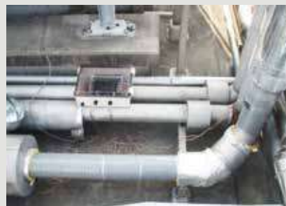
Installation de Vulcan S100
